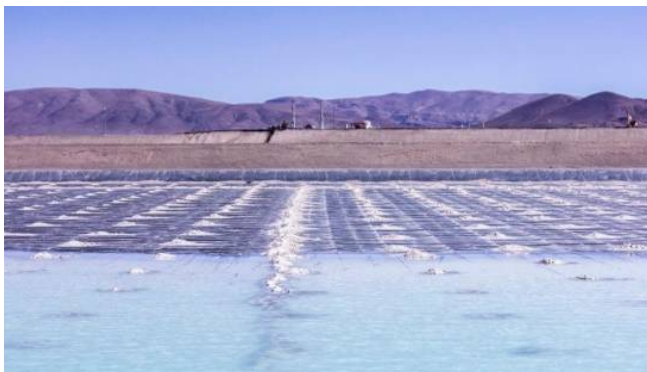
Figure 183: ORE's Olaroz pond system (being filled)
