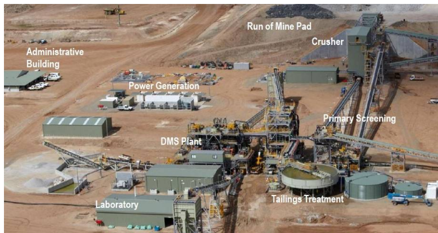
Figure 226: Mt. Cattlin ROM and processing plant
