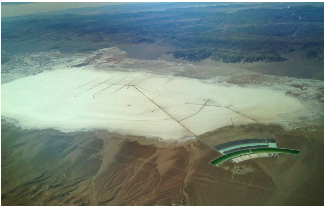
Figure 214: The Olaroz processing plant and pond system (bottom right) and the Olaroz wellfield and salar
