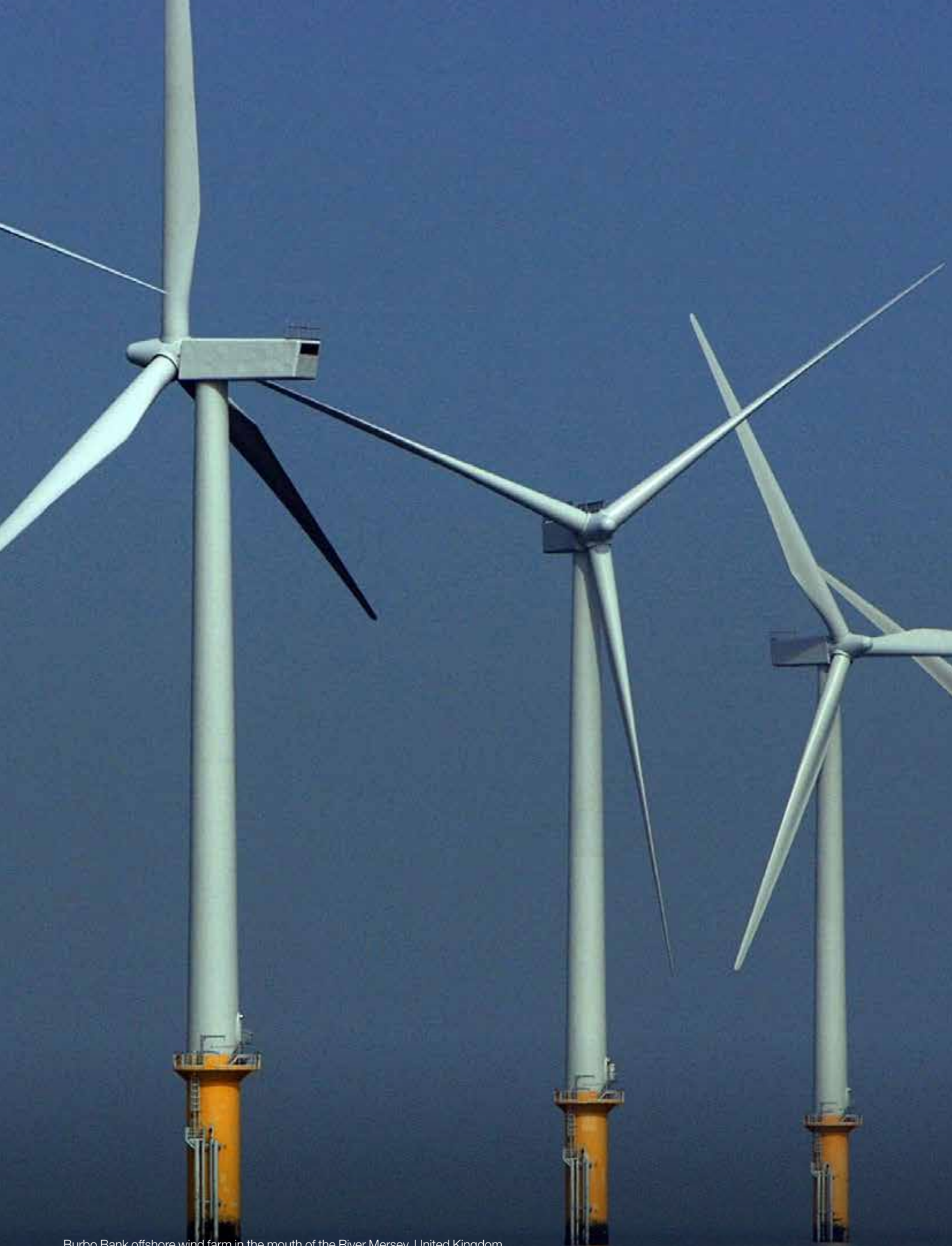
Burbo Bank offshore wind farm in the mouth of the River Mersey, United Kingdom. © Christopher Furlong/Getty Images
