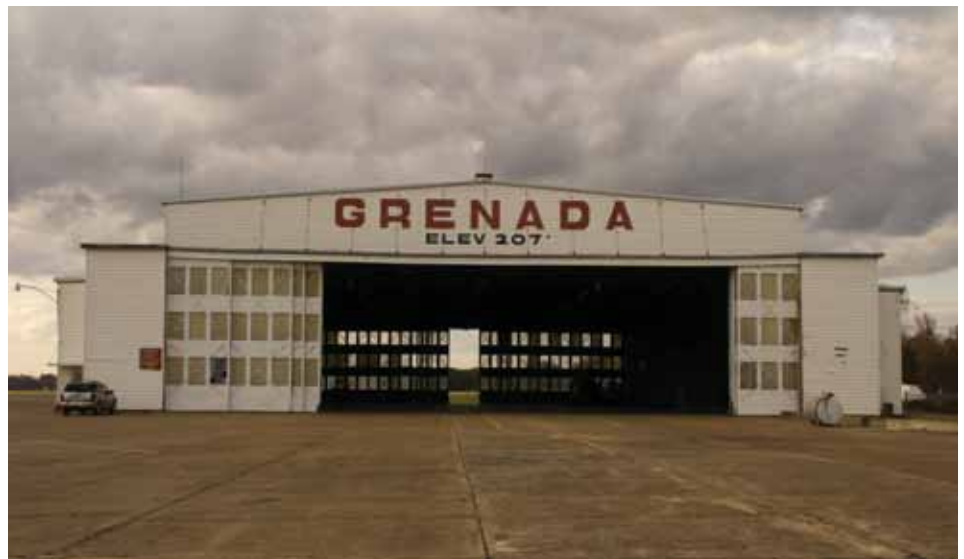
Grenada’s city-owned general-aviation airport includes a wooden structure dating to World War II. One of the three runways is 7,000 feet long and capable of handling big jets. The Mississippi National Guard uses the airport for weekend training exercises, and the Grenada Tourism Commission sponsors aerobatic competitions there.
